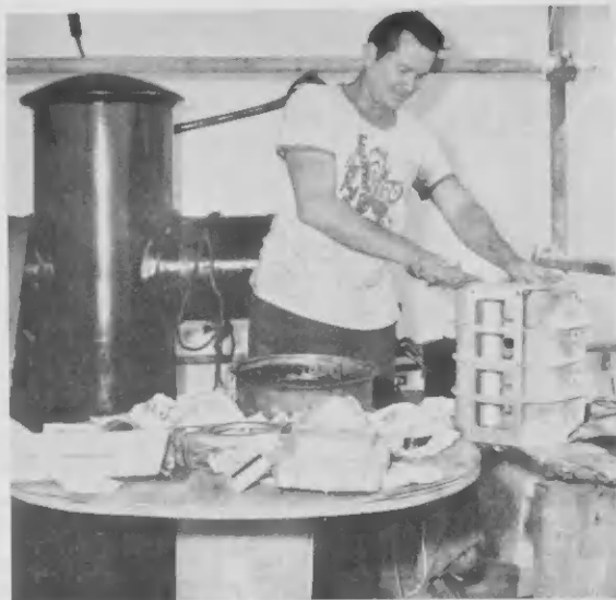
During tug outage, acting tug engineer Pedro van der Linden takes advantage of the situation by overhauling the blower of the auxiliary generator.
